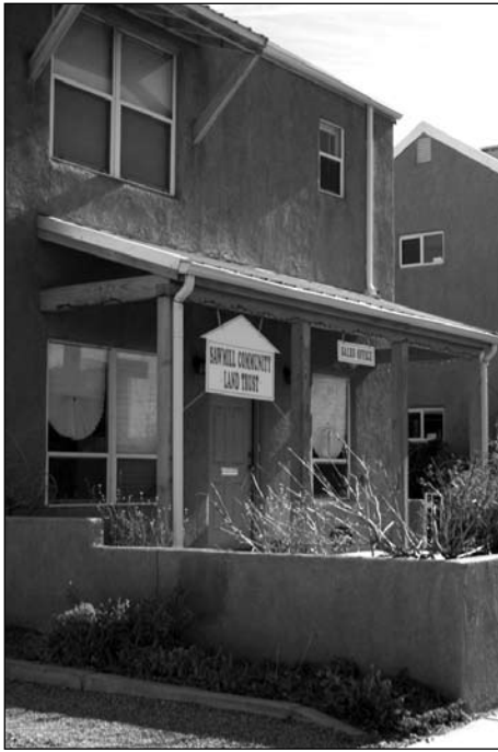
Above and opposite: a large-scale inner-city redevelopment project completed by the Sawmill Community Land Trust in Albuquerque, New Mexico, USA.
