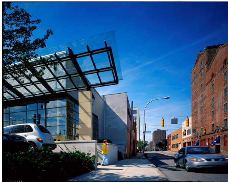
Entrance to Whole Foods parking lot, East Liberty, Pittsburgh
